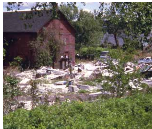
Scenic Hudson removed 75 dump-truck loads of debris from the former junkyard (2001)
